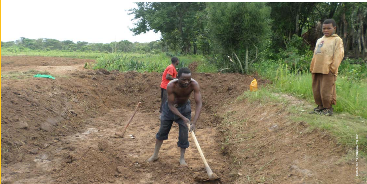
Moving excess silt from pond bottom to the garden.
