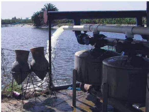
This concrete-lined reservoir for storage of Nile water is stocked with tilapia. The water passes through sand filters (right) before it is pumped into the drip irrigation system.
