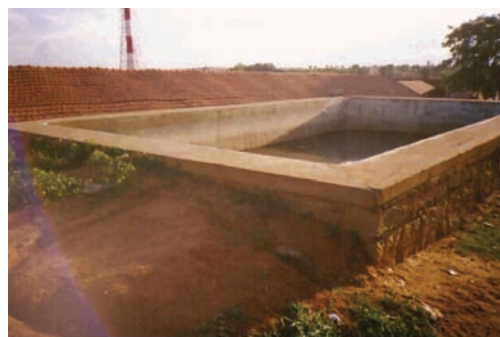
Fig. 2. Bore well water storage pond inlaid with stone blocks
