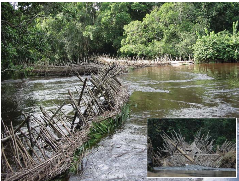
Fig. 6. A fish dam, or alam, constructed on the Fala River, a tributary of the So'o in the central Nyong watershed. Fish migrating upstream to spawn pass over the dam which is submerged at high water. As water levels drop, adult fish returning from the spawning grounds are trapped, while smaller individuals pass through. Inset shows a detail of the chute where fish are stranded. (Photo: R E Brummett.)
