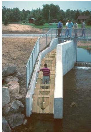
Figure 69: Denil fish pass (Trout Creek, USA). Photo Michigan DNRE.
