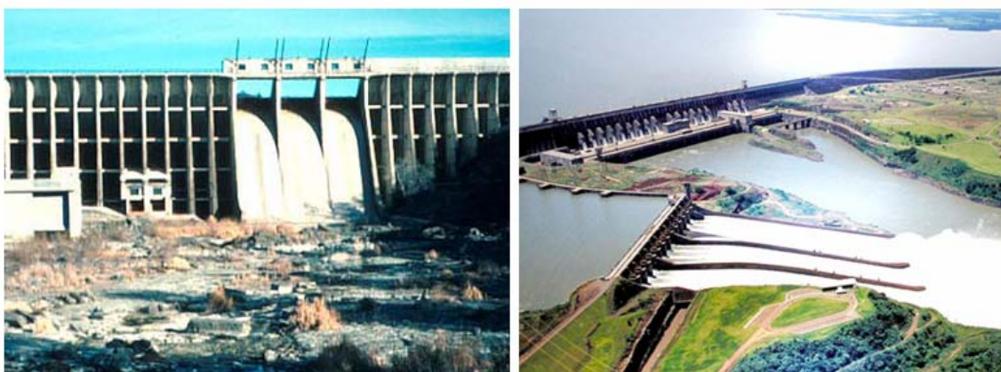
Figure 61: Two different types of spillway designs. Photos: Matt Kondolf and Itaipu Binacional
