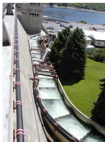
Figure 66: Pool fish pass of the Grand Coulee dam (USA). Photo Erin A. Barnes.
