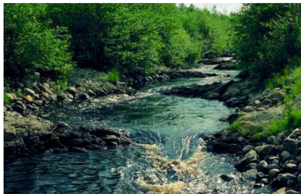
Figure 65: Natural bypass channel created on the Siikajoki River (Finland) to overcome a 4m high dam. Photo G. Marmulla.
