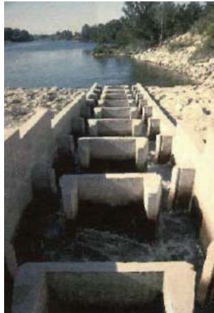
Figure 67: Vertical slot fish pass on the Gardon River (France). Photo M. Larinier.
