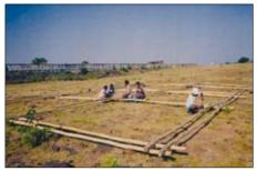
Fully grown, cured bamboo poles at least 7.5 metres long and 8-9 cm in diameter at the base are best suited to make the frame. To make a battery holding eight cages, each measuring  $15 \text{ m}^2$ , the battery should be 13.75 metres long and 11.05 metres wide. To make such a frame, 32 bamboo poles are required for the top frame and 24 for the lower frame.
