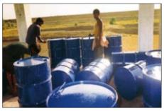
Floats are painted with acrylic paint and fastened with the frame with glazed iron (GI) wires.
