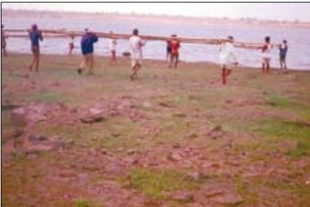
Four poles are used to make one long side of the rectangle. Two poles are placed on the ground with their tip portions overlapping to make their combined length at least 14.5 metres. Six such lengths are made for the two long sides and the central divider. Each long side and the central divider consists of two such 14.5-metre lengths placed parallel 35 cm apart.
