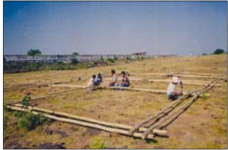
Fully grown, cured bamboo poles at least 7.5 metres long and 8-9 cm in diameter at the base are best suited to make the frame. To make a battery holding eight cages, each measuring 15 m<sup>2</sup>, the battery should be 13.75 metres long and 11.05 metres wide. To make such a frame, 32 bamboo poles are required for the top frame and 24 for the lower frame.
