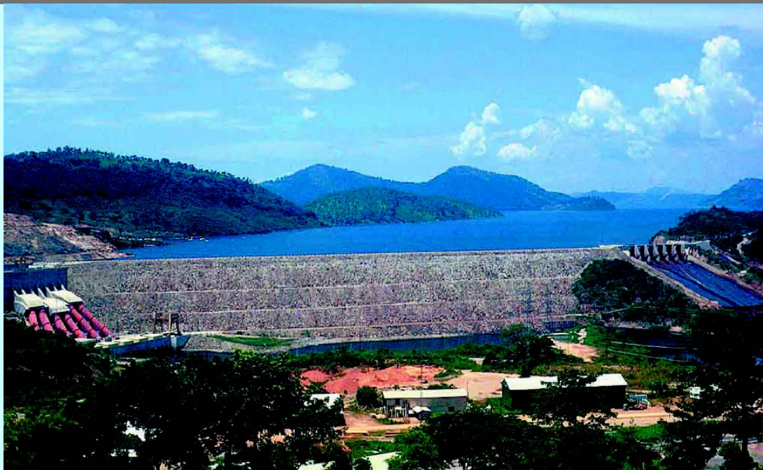
Photo: The Akosombo dam
