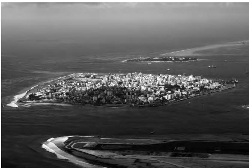
Malé, the capital of the Maldives, is one of the most densely populated islands in the world with more than 80,000 people living within 2 square kilometres. The tsunamis flooded some of the island and damaged parts of the seawall, buildings and vehicles parked on the roads (photo from Hussein Zahir).
