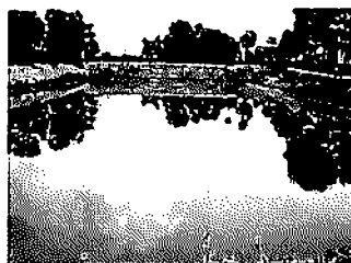
A completed pond after vegetation removal, and slope repair.
