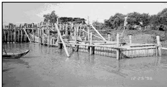
Figure 3. A freshwater estuary barrage and rectangular trap in Kandal Province
