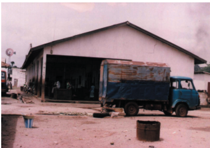
The fish landing and marketing facilities at the Gunjur CFC.
