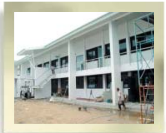
The new HQ : building in progress
