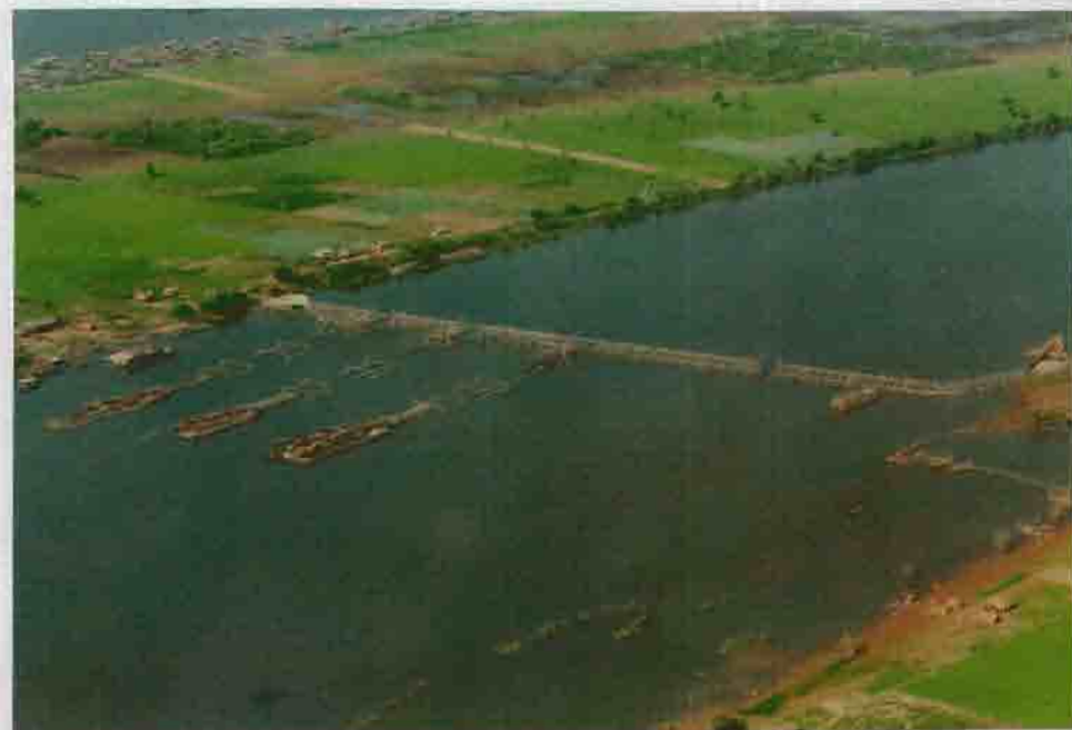
Fig. 3. The barrage across a branch of the Tonle Sap River near Kampong Chhnang town is part of a fishing lot concession. Three openings admit migrating fish through a passageway made of netting into the fish pens. The other opening is navigable for small craft. Fishery regulations do not permit the blocking of all river branches. Operational from November to May.
