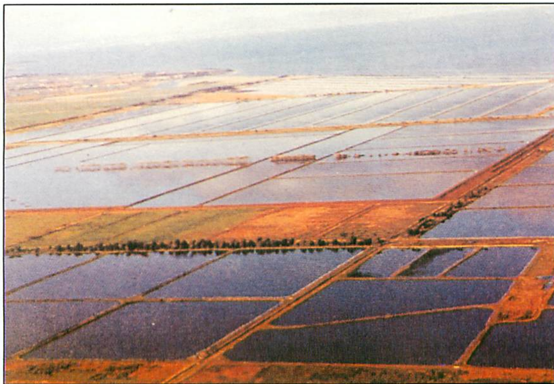
Werribee sewage treatment lagoons (WSTL) is the largest treatment plant in Australia. Zooplankton grow in abundance in the last stage of water purification process and remove phosphorus and nitrogen from the system. One hundred tons of wet zooplankton contain about 100 kg of phosphorus and 1 t of nitrogen.
