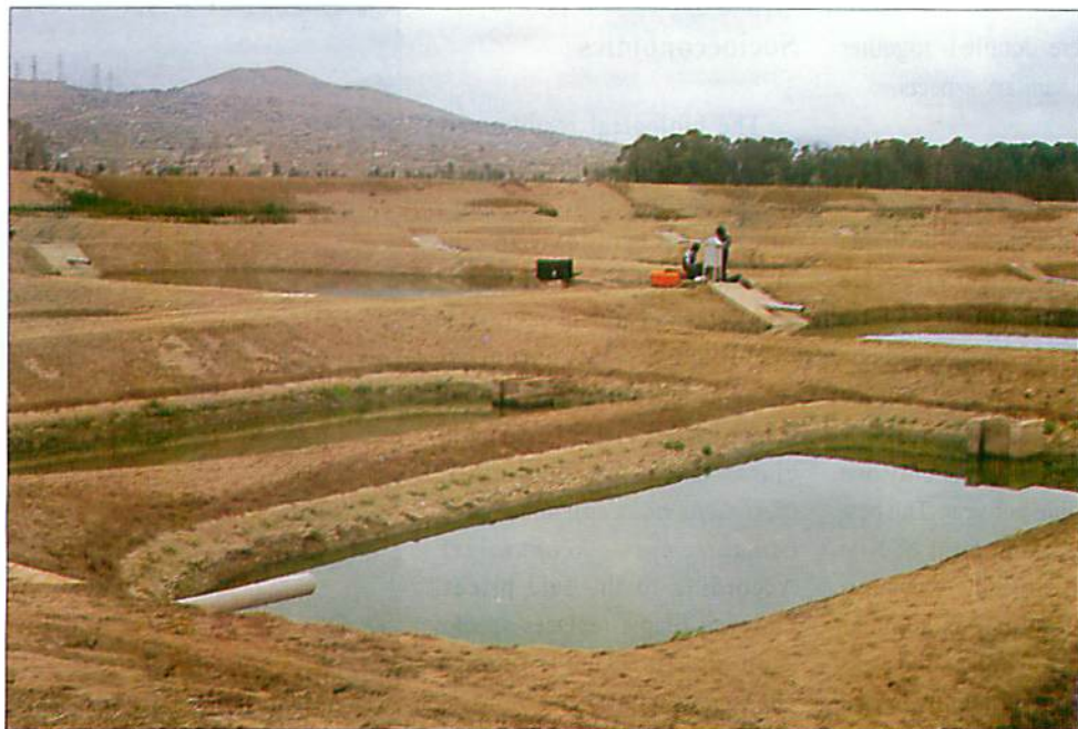
Experimental fishponds built within the municipal wastewater treatment plant area consisting of stabilization ponds. The township of San Juan is visible in the background. ALL PHOTOS BY MARK PREIN, ICLARM.
