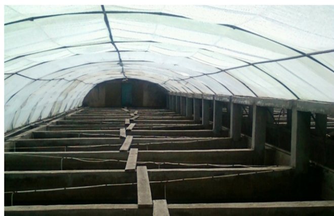
Fig. 3. Heated greenhouse hatchery (concrete tanks under a greenhouse tunnel equipped with a water heating system).
