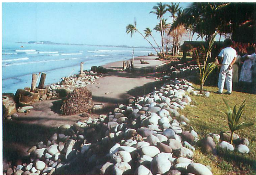
Plate 4. Revetments protect this beach resort in Lingayen Gulf, Philippines.
