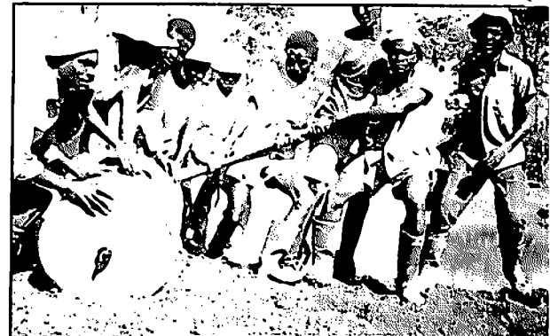
"Unity is strength" demonstrated by the trainees pushing a roller to compact the embankment of a pond.
