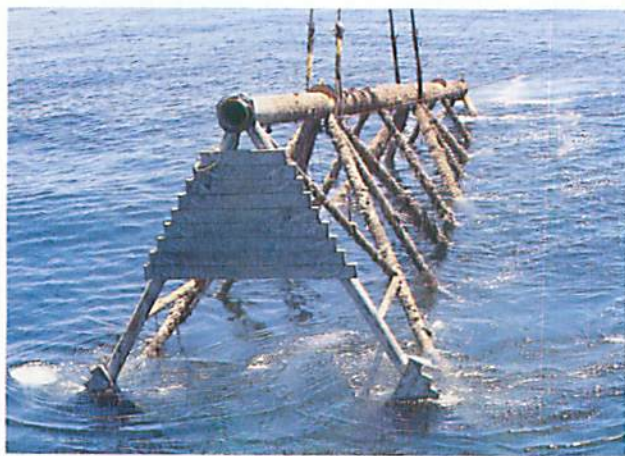
Plate 5. An obsolete oil-well jacket being set into place in Brunei Darussalam. (Photo by M.W.R.N. De Silva.)
