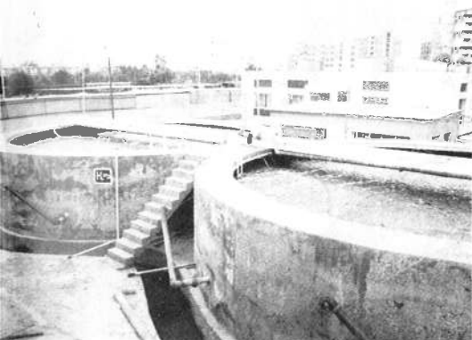
250-m 3 tanks used for tilapia culture.
