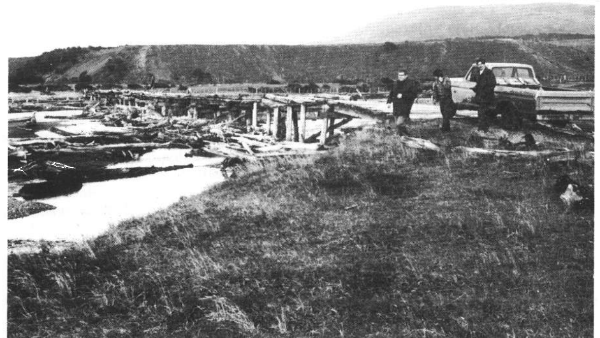
Figure 29. Brunswick Peninsula; Rio el Canelo bridge.
