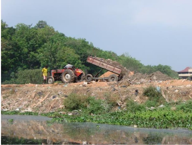
Photo 5.2. A wetland area being reclaimed using solid waste in Colombo.
