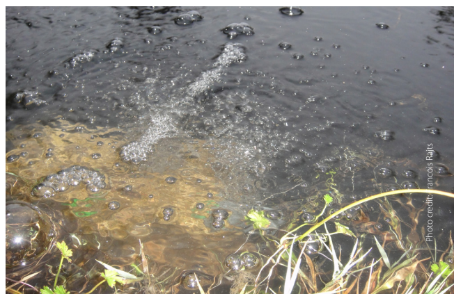
Plate 6. An air diffuser pond/tank aerator in operation.
