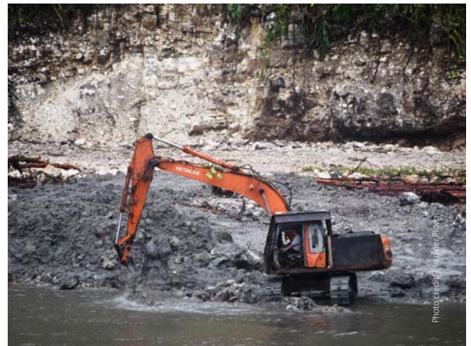
Plate 6. Log pond construction on the east coast of Malaita.
