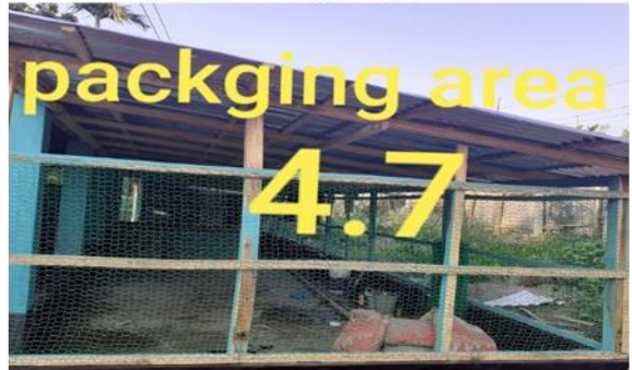
Renovate the product loading packaging area:
