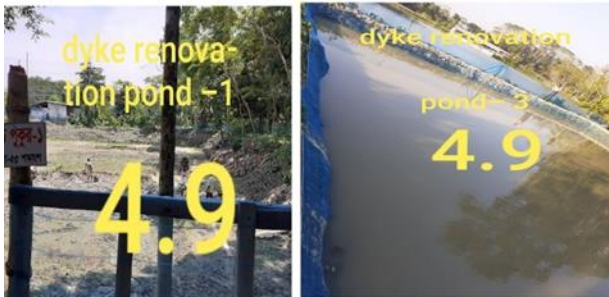
Sludge removal and pond bottom/dyke renovation:
