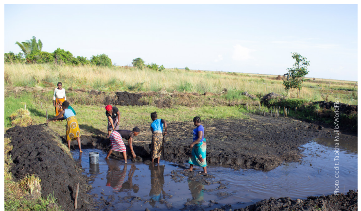
Pond construction by Nsombo women in Luwingu, Northern Province, Zambia.
