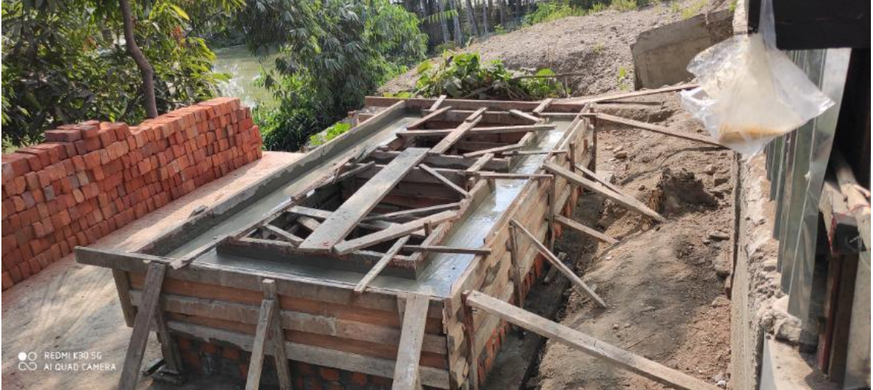
Figure 6: Formwork mould for pouring the concrete mix into
