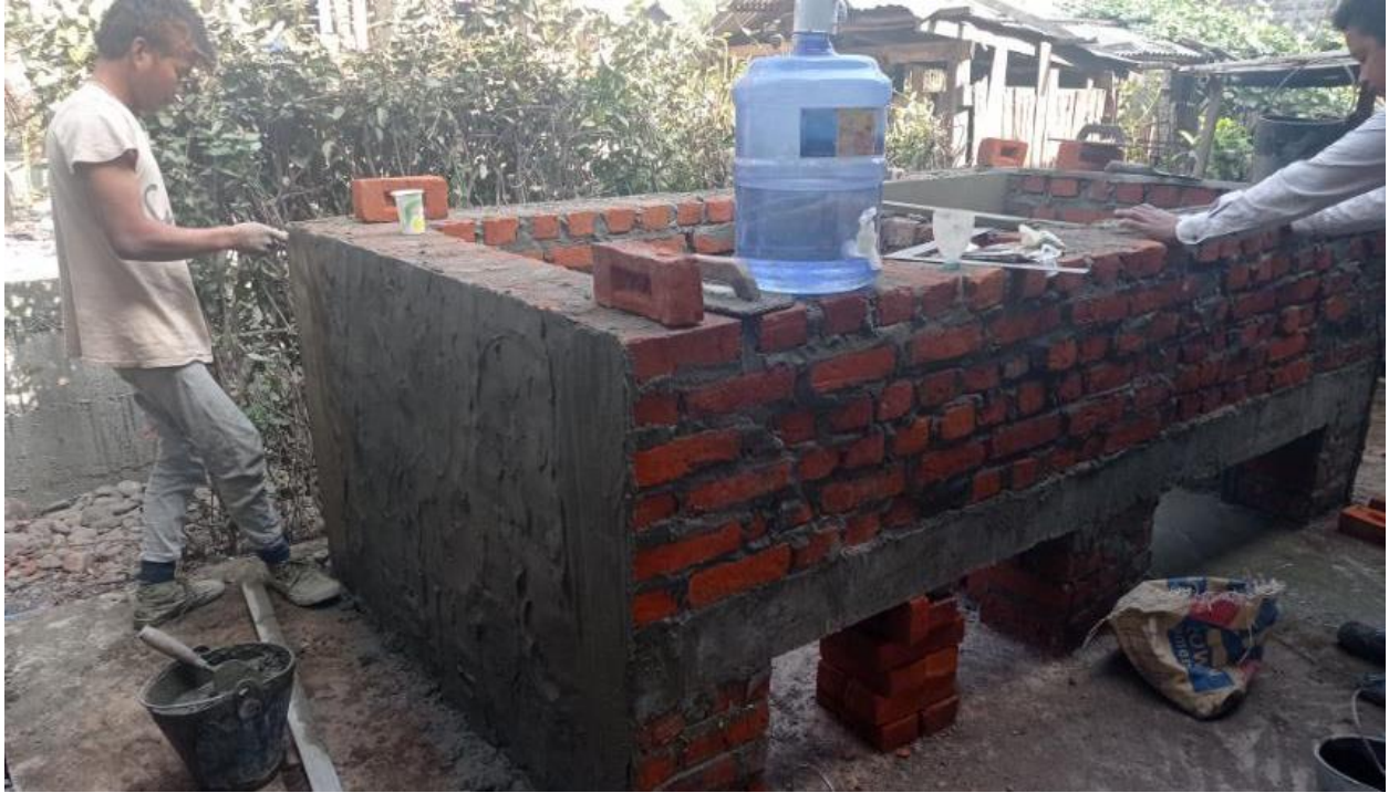
Figure 9: Plastering the walls of the kilns
