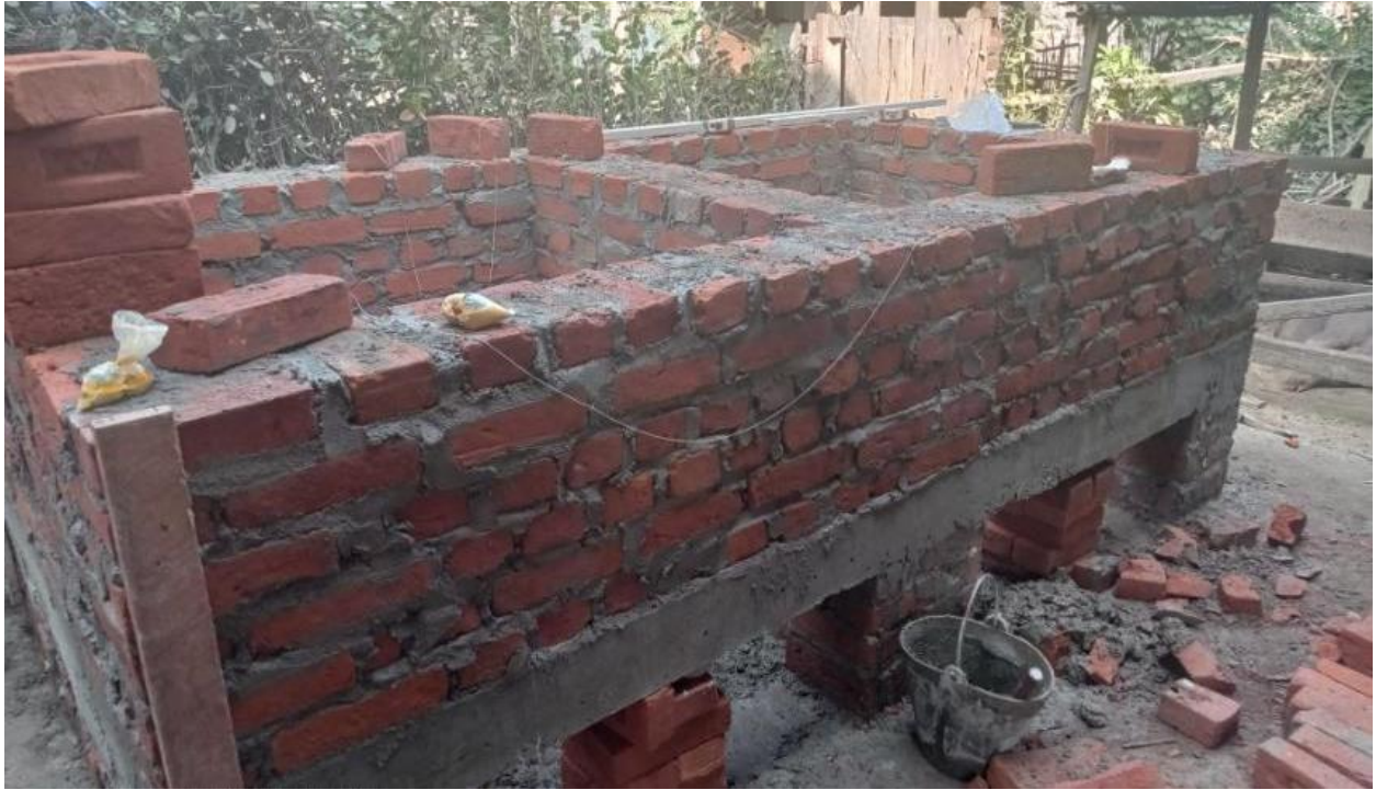
Figure 7: Continue the brick works on top of the concrete reinforced beam
