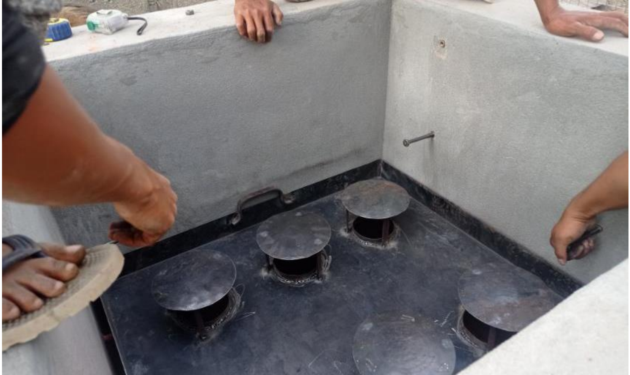
Figure 11: Confirm that the oil tray can be moved smoothly lowered into position inside the kiln chamber
