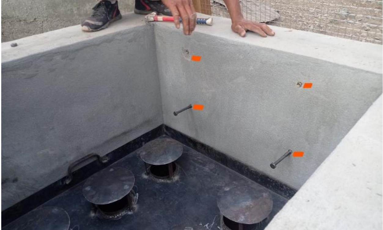
Figure 13: The position of the smoking racks can be easily adjusted by having iron rebar or iron bolts inserted at different heights in the kiln wall
