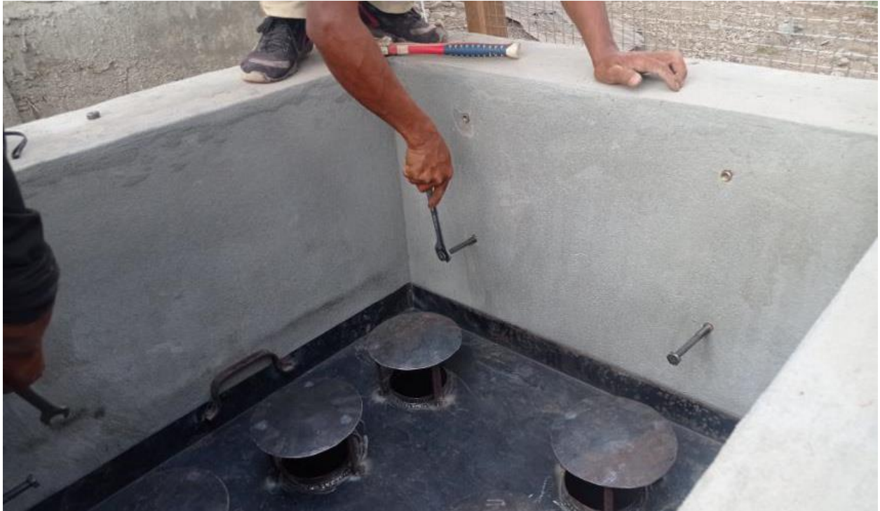
Figure 15: A piece of rebar or iron bolt can be used to fix the position of the smoking racks
