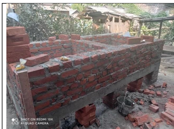
Daw Vuli, Pyin Khone Lay Village Kale Township
