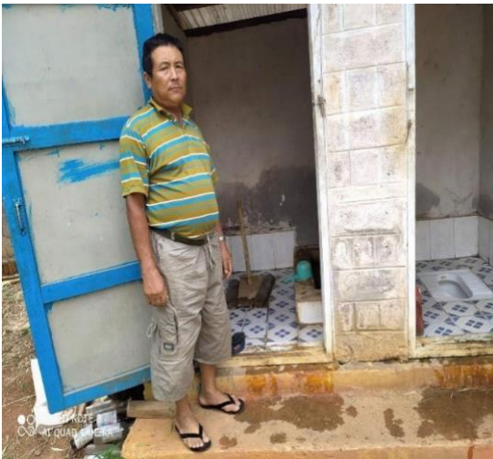
Photo 1. Pour flush toilet in an SSA household in Taunggyi.
