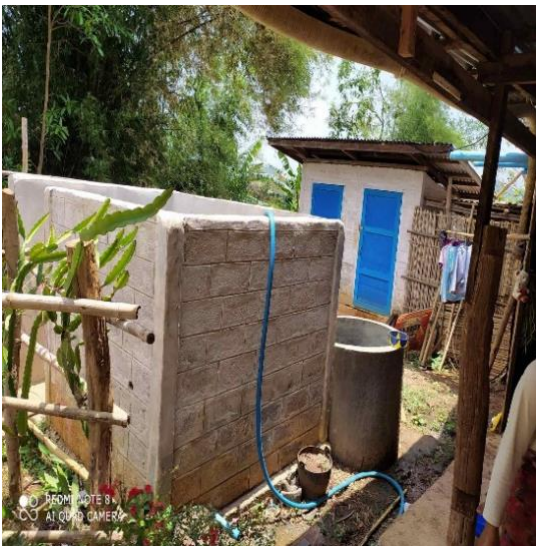
Photo 3. Water tank near the toilet.
