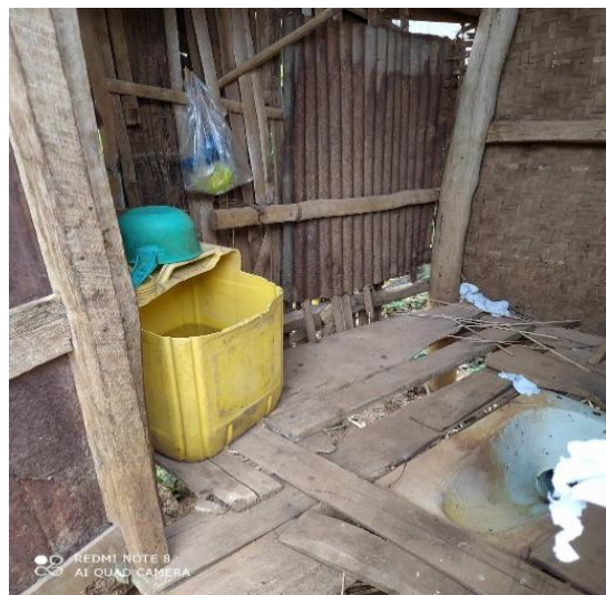
Photo 6. A toilet with a plastic toilet bowl.
