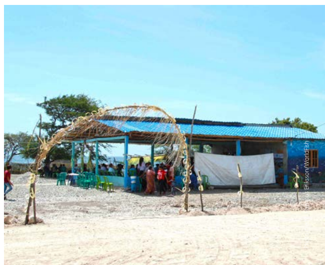
The completed Ililai Fish House.
