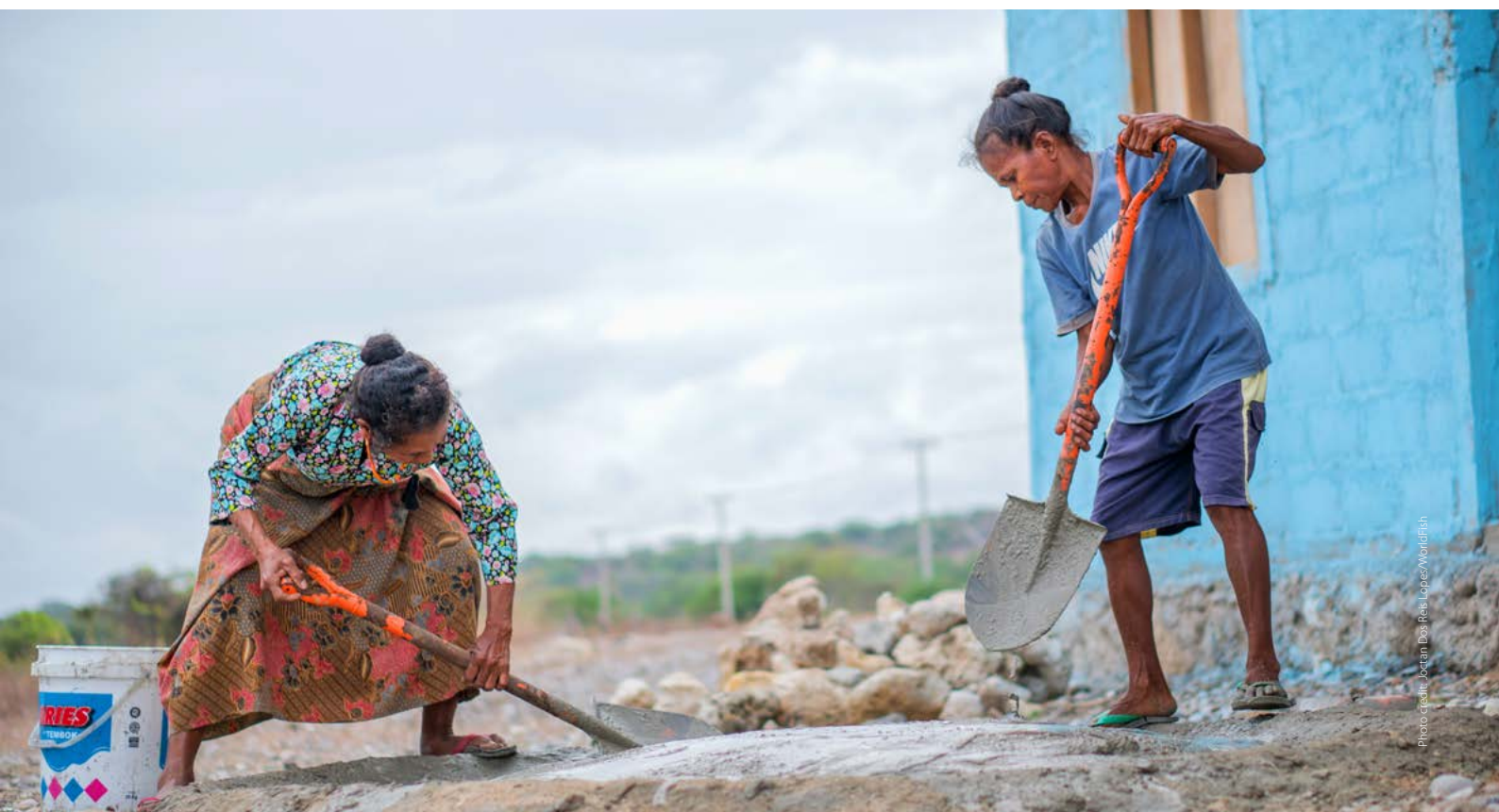
Ililai women mixing concrete to build the floor of the Fish House.
