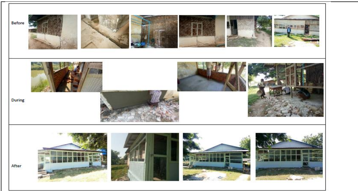
Photo 04. Renovations at the DoF Nad Yan Kan satellite GIFT hatchery facility.
