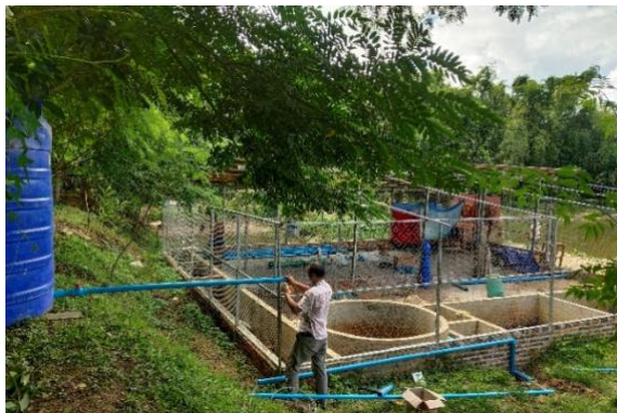
Figure 13. Ongoing renovation of a hatchery in Eastern Shan Township.
