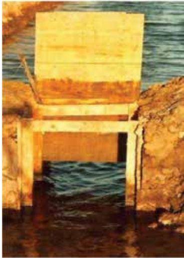
Figure 34: Monk with filter to prevent predators entering in the Artemia pond
