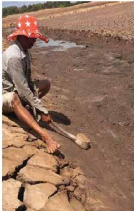
Figure 29: Dike compaction
