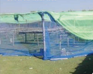
Photo 1. Bamboo structure covered with net
