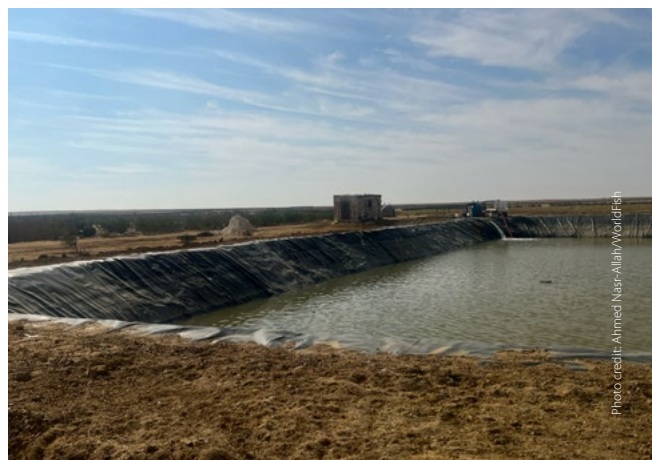
Plate 1. Rectangular polyethylene-lined pond.
