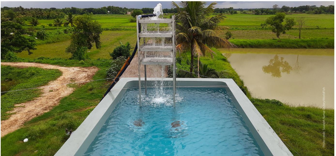
Plate 8. An aeration tower installed within the overhead water reservoir tank in a hatchery.
