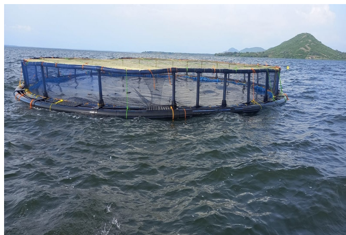
Figure 9. Locally fabricated 20 m-diameter HDPE cage in Lake Victoria, Kenya.
