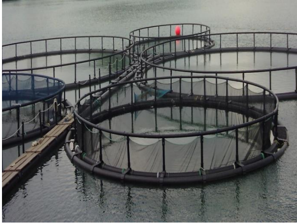
Plate 2.1 Circular cages made of HDPE pipes
