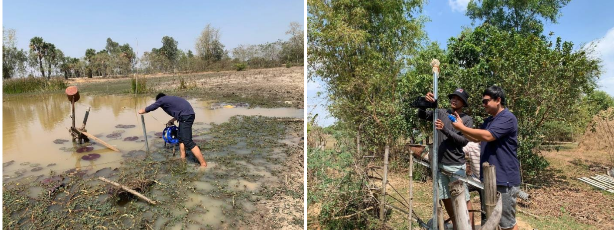
Figure 4: Installation of water level sensor and rain gauge station
