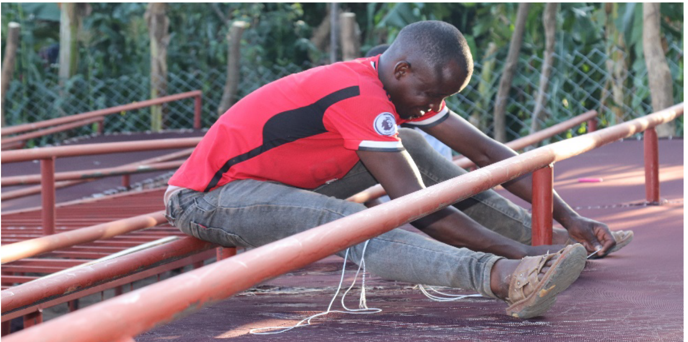
Figure 3. The contractors and some community members during the construction phase.
