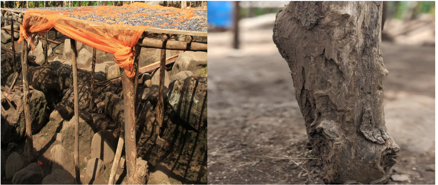
Figure 2. The old drying racks made of wooden poles were eaten by ants, reducing sustainability in climate change.
