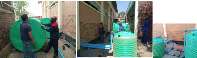
Pipe work and installation of sand filter and tanks for mechanical and biological filtration
