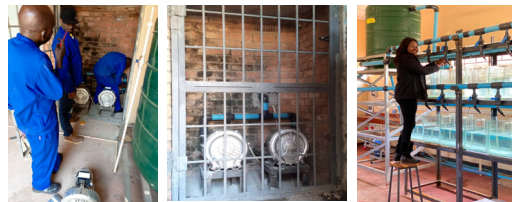
Securing area and installation of air blowers to supply oxygen to fish tanks and biological filter
