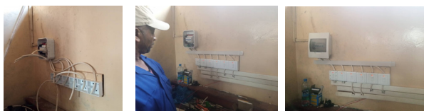
Electrical switch board installation (control of water heaters, air blowers, water pumps)
