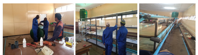
Pipe works to ensure indoor water supply to aquarium tanks
