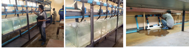
Testing of water flow system and works on linkages
