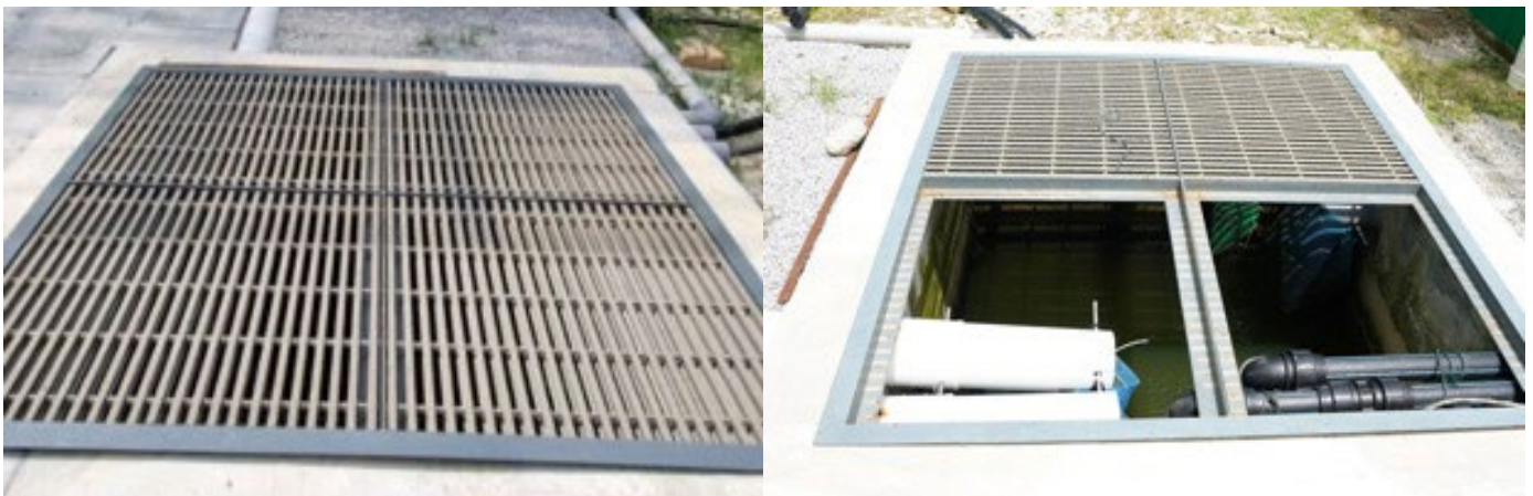
Plate 12. Fitting the main sump tank with a UV will kill pathogens before discharging effluent.
