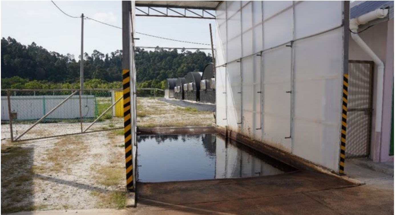
Plate 10. A drive-thru wheel bath at the entrance of the hatchery can mitigate the risk of potential pathogens.
