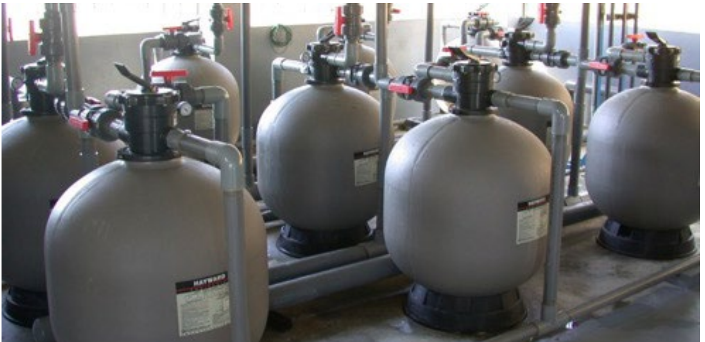
Plate 7. Treating the water supply with a sand filter can remove organic matter and possible pathogens.
