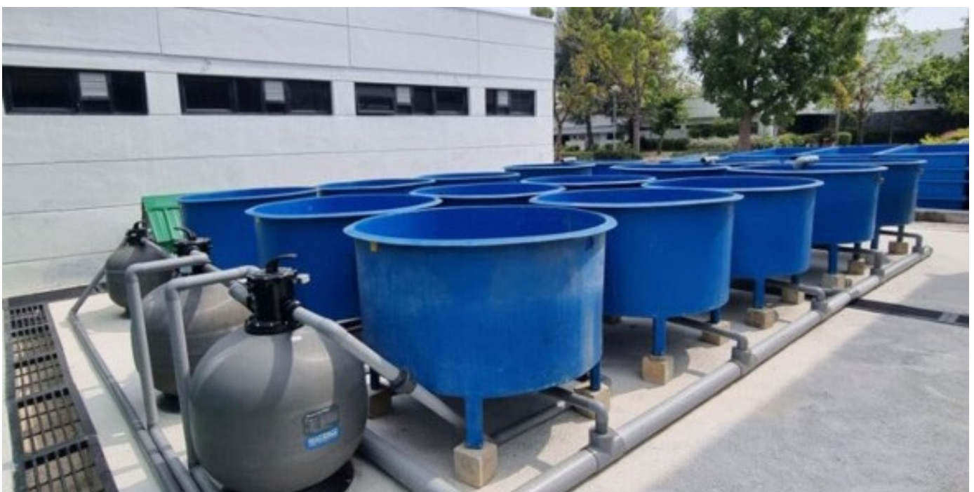
Plate 13. Hatcheries should have a wastewater treatment section with settling tanks and a sand filter.
