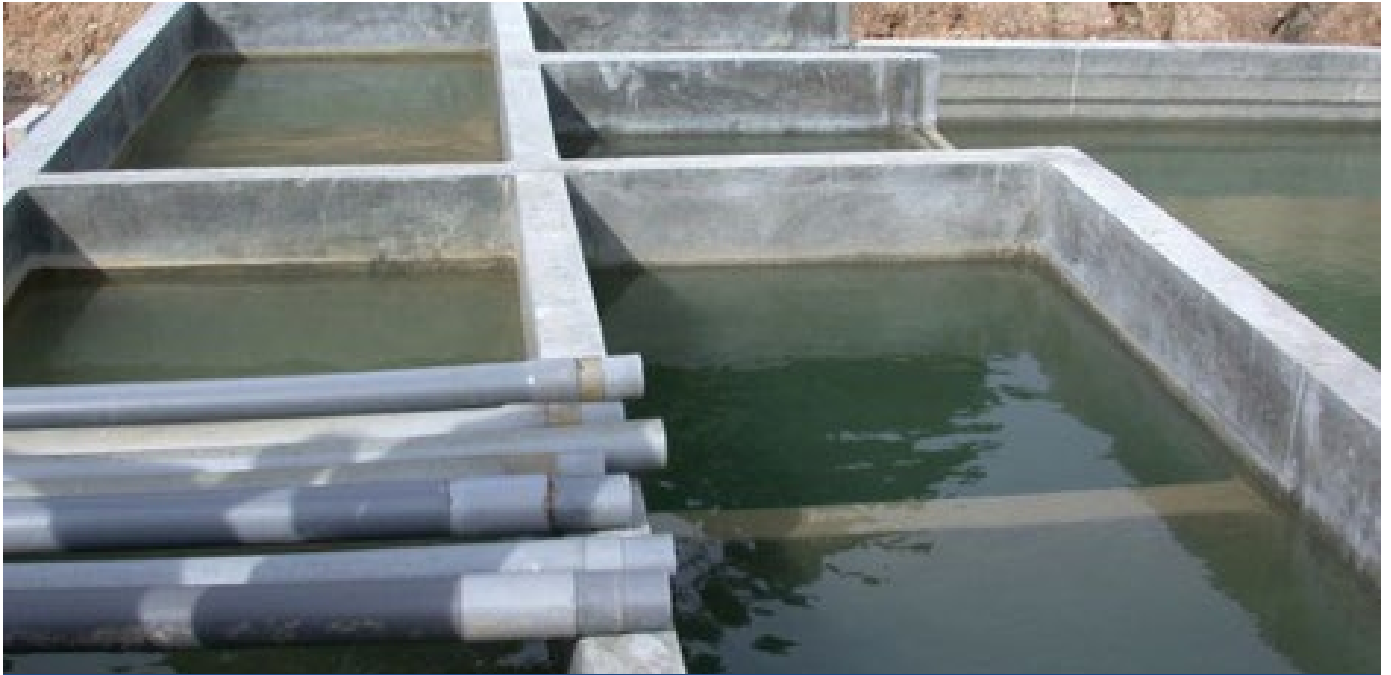
Plate 6. Using comprehensive water filtration across multiple chambers can eradicate organic matter, aquatic predators and potential pathogens.
