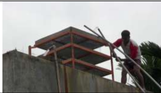
Setting water tower in a hatchery
