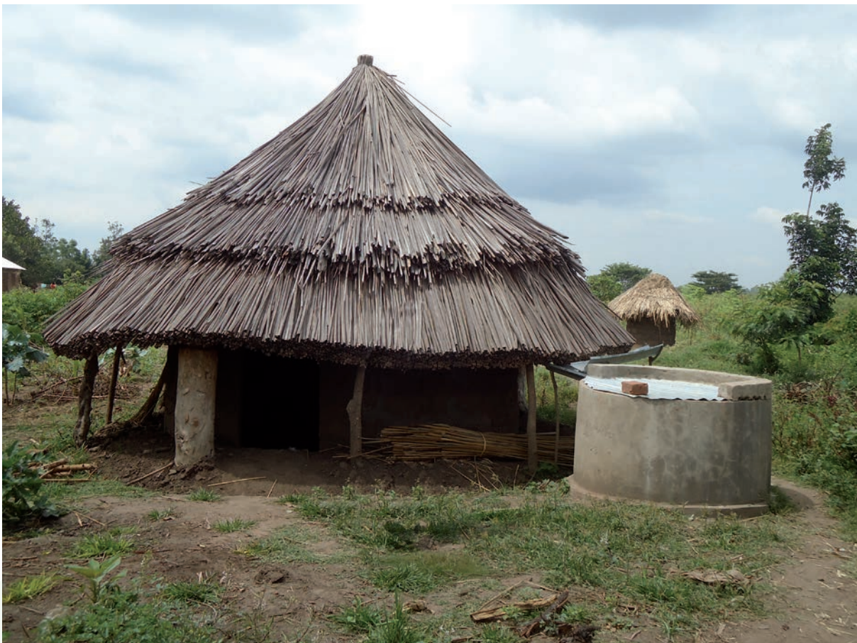
Above: Rain water is harvested from papyrus roof and stored in concrete tanks for use during periods of scarcity
