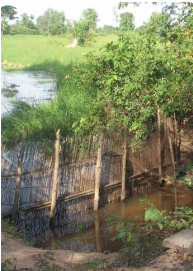
Bamboo fence blocking fish from migrating out of the refuge pond before flooding.
