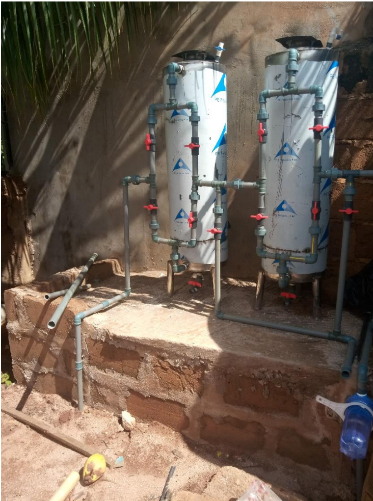
Image 14: Water purification units at Uvwie in Delta State
