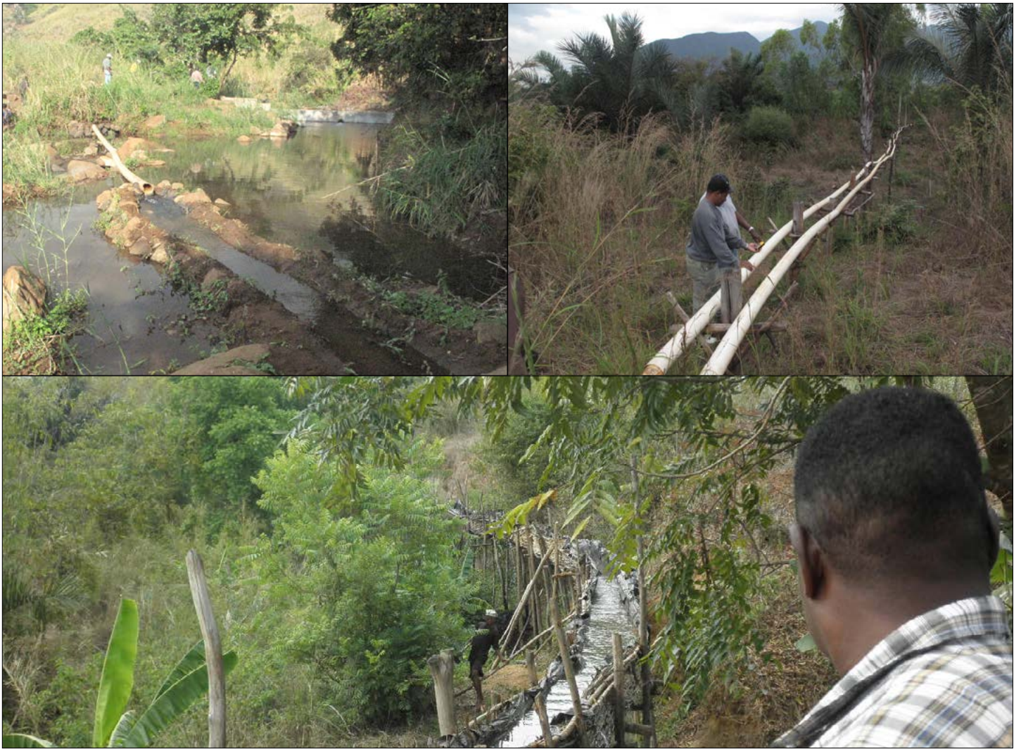
River diversion and conveyancing
