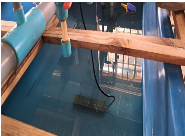
Plate1 Installed water tank heaters for improved heat conservation NAC in Domasi, Malawi.
