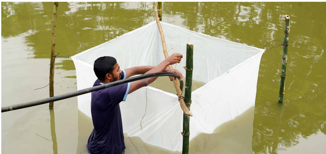
Photo 8. Installation of 100-micron monofilament mesh to filter water prior to use for hatchery operation. Photo credit: Harun Or Rashid, WorldFish.
