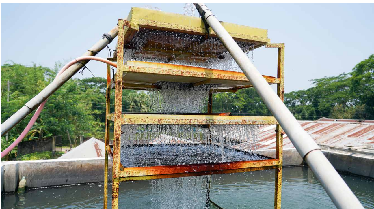
Photo 9. An aeration tower in an overhead water reservoir tank at a hatchery. Photo credit: Harun Or Rashid, WorldFish.
